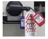
Locks and tags both are required if they can be installed on circuits with an operating voltage of 50 volts or greater. Lockout is only one step in establishing a safe work condition.
